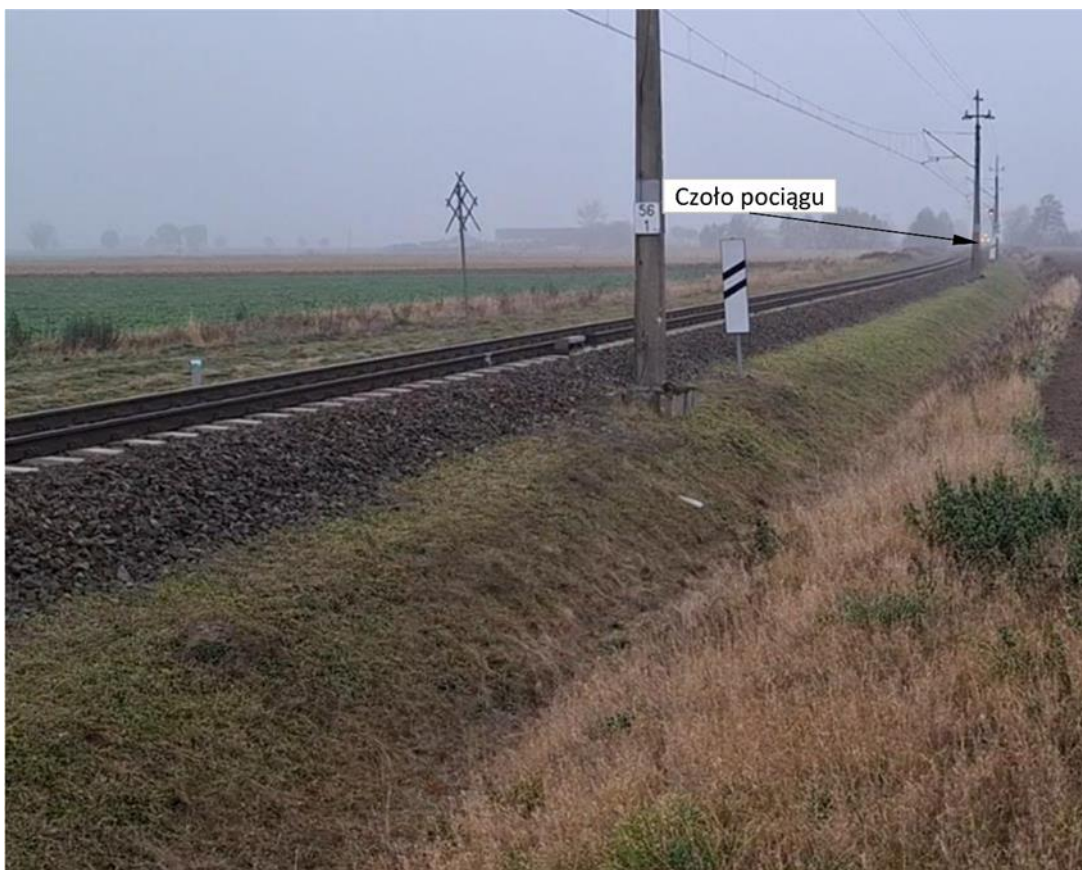
Photo 9 – Visibility of the train front from the pedestrian’s position (source: GDPWK)
