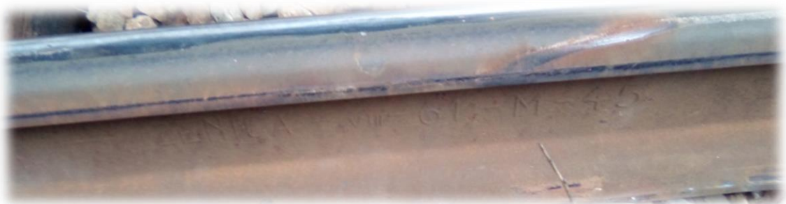
Figure 4.2.8.1: Appearance of the rail “S45” ZENICA VIII-61
