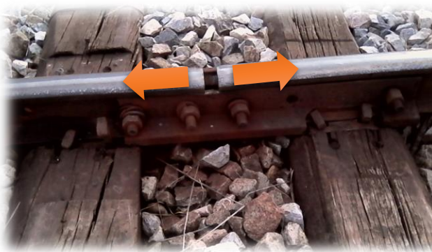
Figure 4.2.10.5: Rail-floating joint connection
