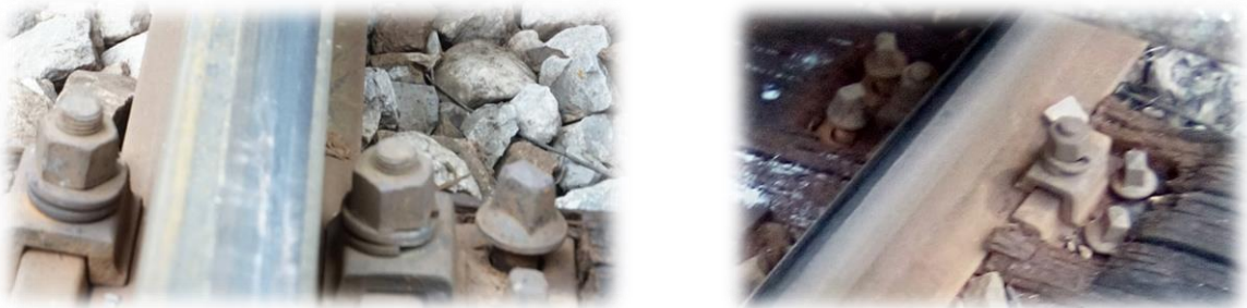
Figure 4.2.10.4: Rail-sleeper connection with an underlying fastening plate and tirphones
