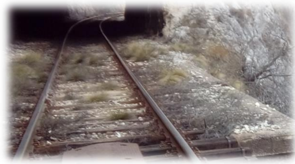
Figure 4.2.8.6: Appearance of the ballast
