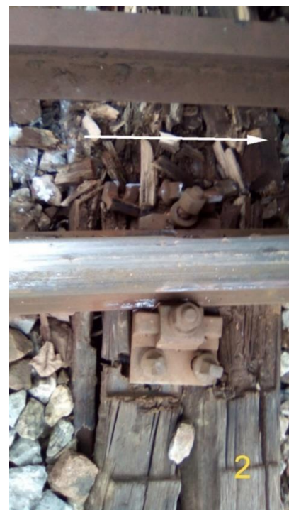
Figure 4.2.1.2: First traces of damages from the entered wheel on the inner rail
