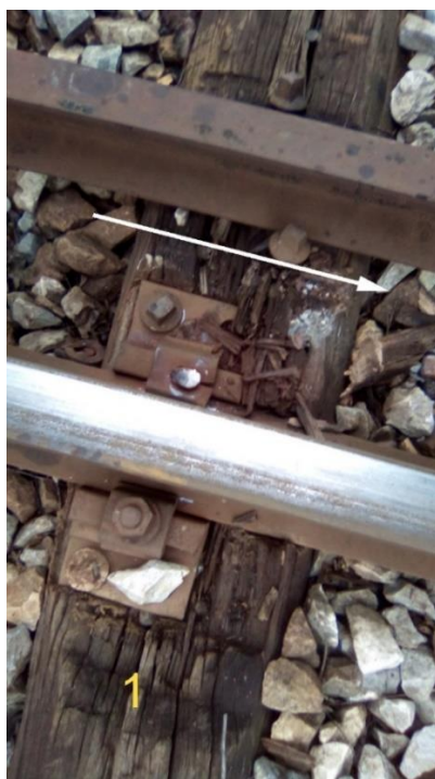
Figure 4.2.1.2: First traces of damages from the entered wheel on the inner rail
