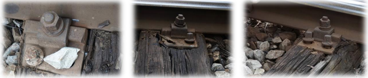
Figure 4.2.8.2: The depiction of rail fastening with tirphones
