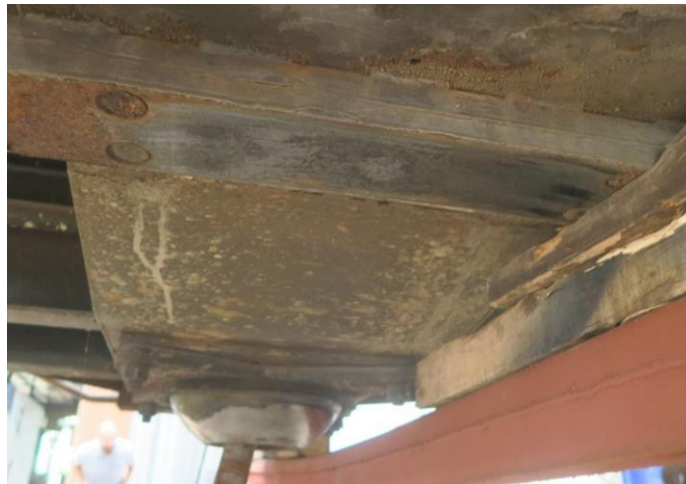
Figure 4.2.6.2: The condition of the upper center bowl and side bearers on wagon No. 33 87 7814 136-0 at housing 7 and 8
