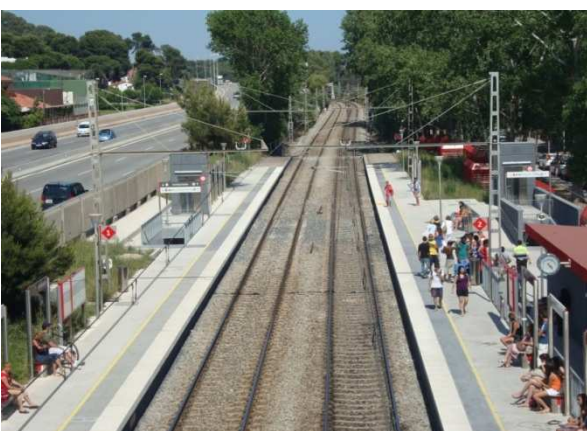
View of the Platja de Castelldefels halt (source: CIAF)
