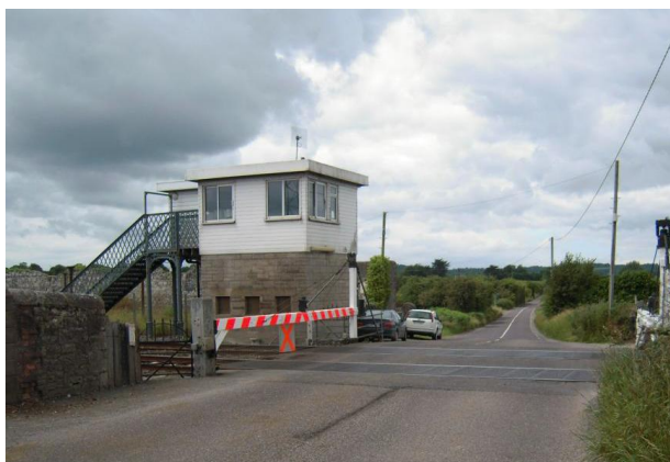
Figure 10 – Level crossing XC219
