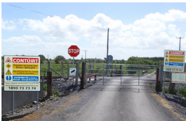
Figure 12 – Level crossing XM250
