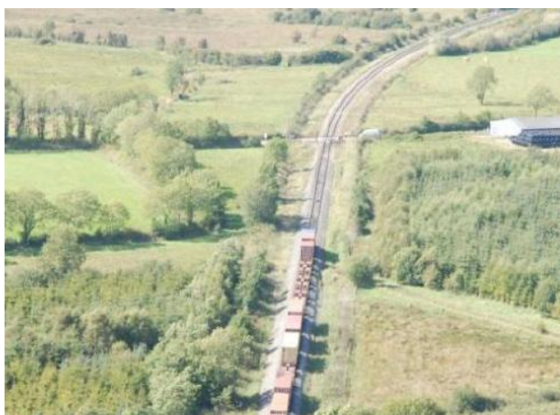
Figure 11 – Level crossing XM096
