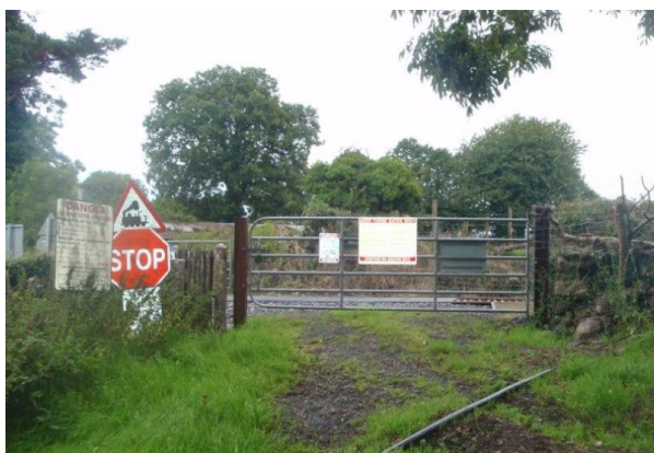
Figure 9 – Level crossing XE039
