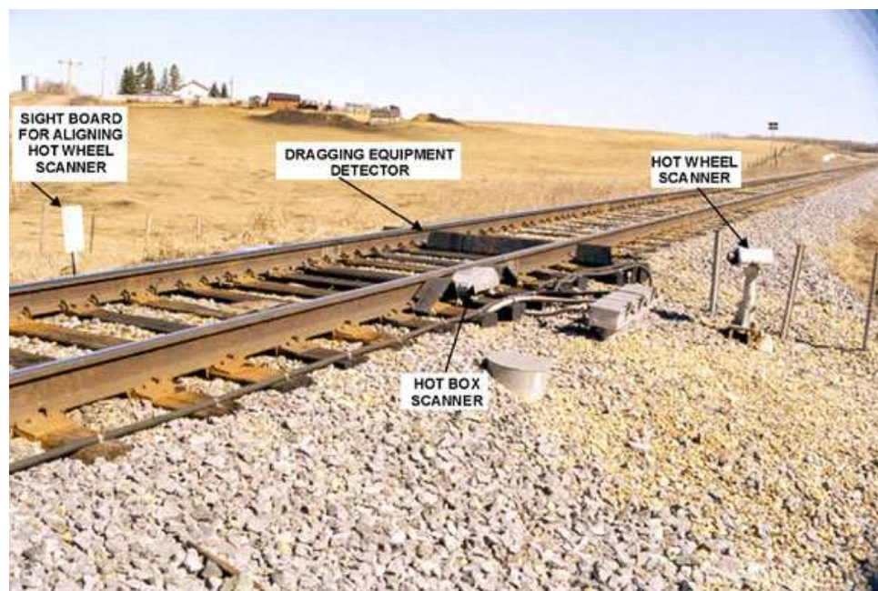
Figure 9: Typical US derailment and dragging object (and other) detectors 10
