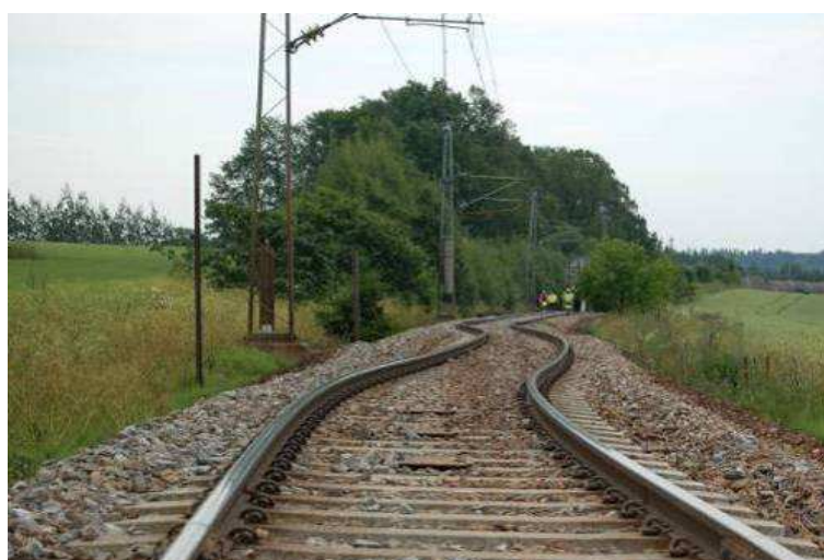
Figure 5: Example of a Heat Buckle 8
