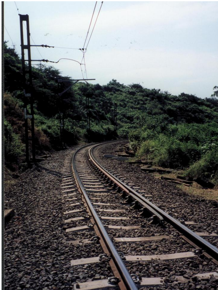
Figure 2: Example from RSA showing check rail installation in curved track
