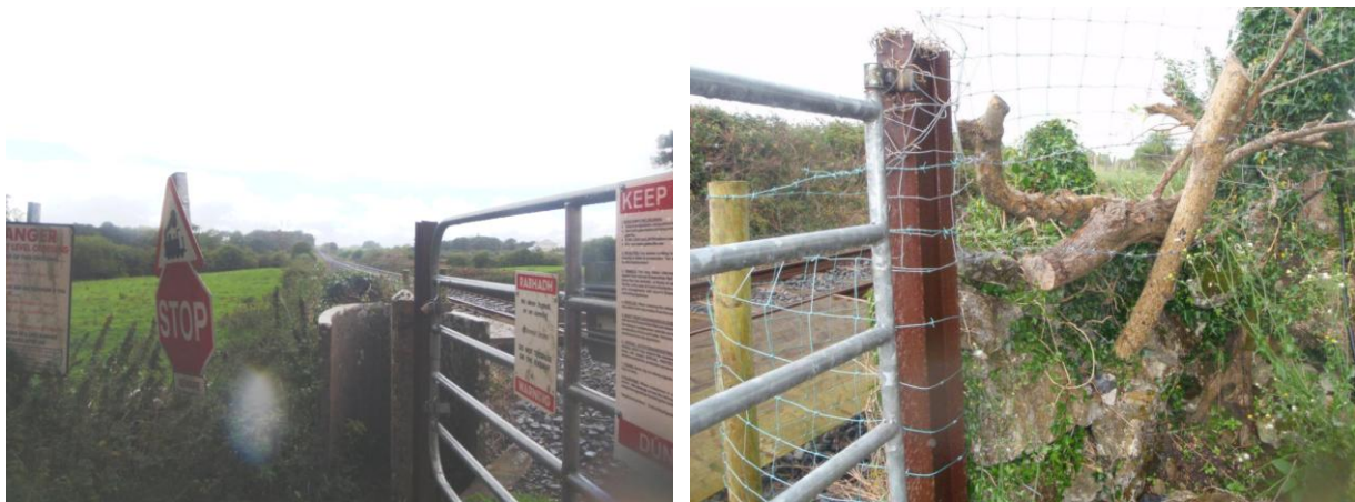
Photograph 4 – Down side view in Down direction Photograph 5 – Down side view in Up direction
