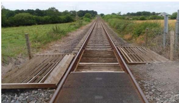
Photograph 2 – Approach from Down direction
