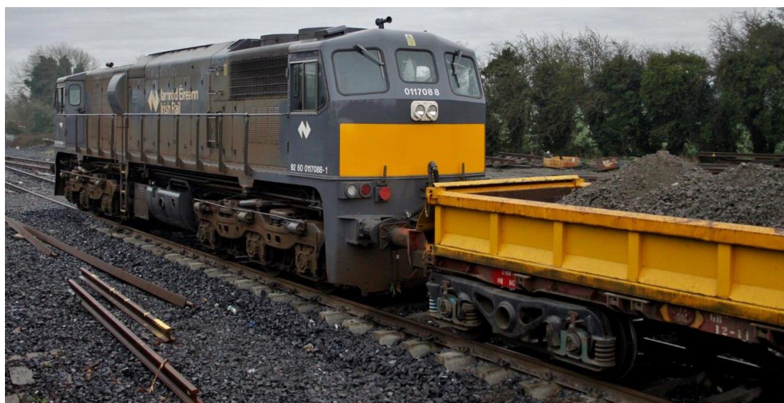
Figure 27 – Locomotive with Spoil Wagons
