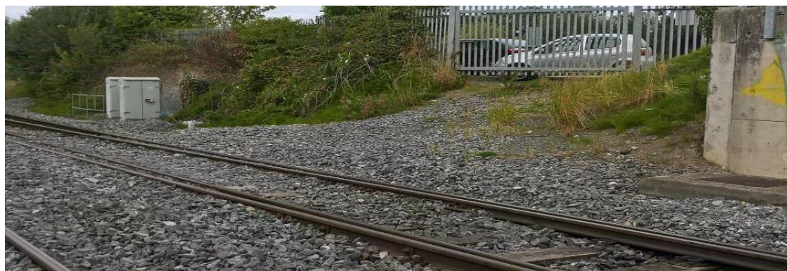
Figure 33 – Ballast Pad (for on-tracking & off-tracking RRVs)
