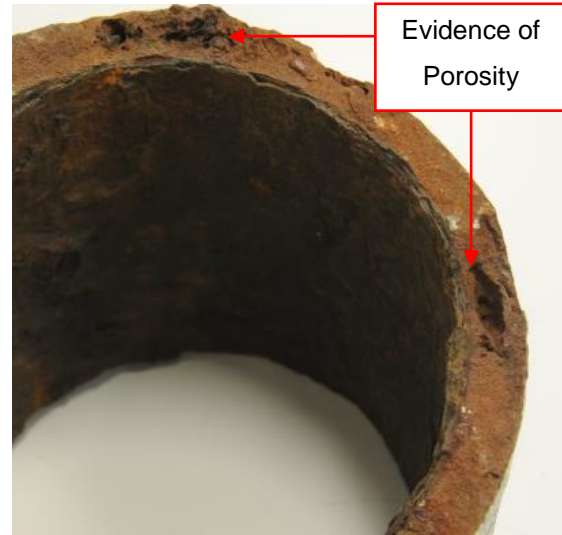
Figure 19 – Areas of porosity in column 16
