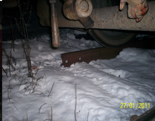
Fig.4 the 2 missing rail coupons on the avoidance line
