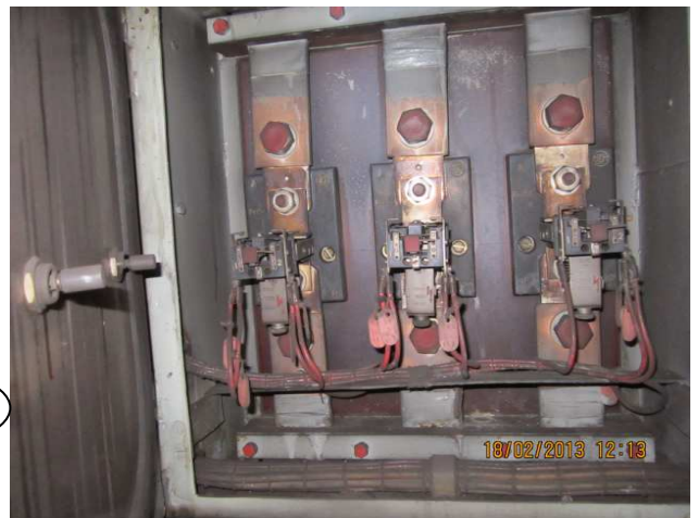
Photos no. 7 and 8 Maximum current relay
