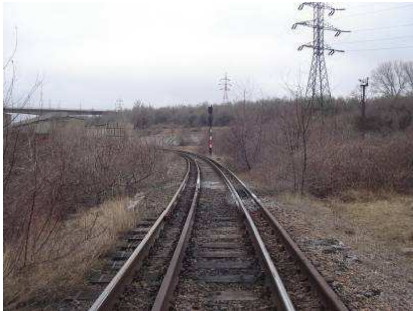
Photo no. 1 The place where the accident occurred
