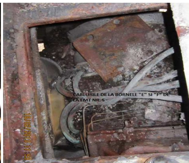
Photo no. 3 The force cables from the EMT no.4 and 5
