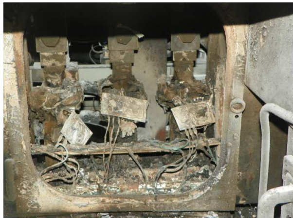
Fig.16 Cofret rele maxime de curent poz.54.1-3
