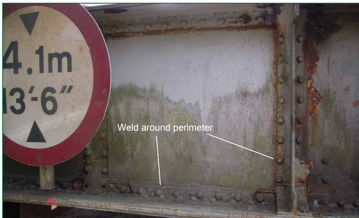
Figure 19: Repair plate welded to web panel 5 of the east main girder
