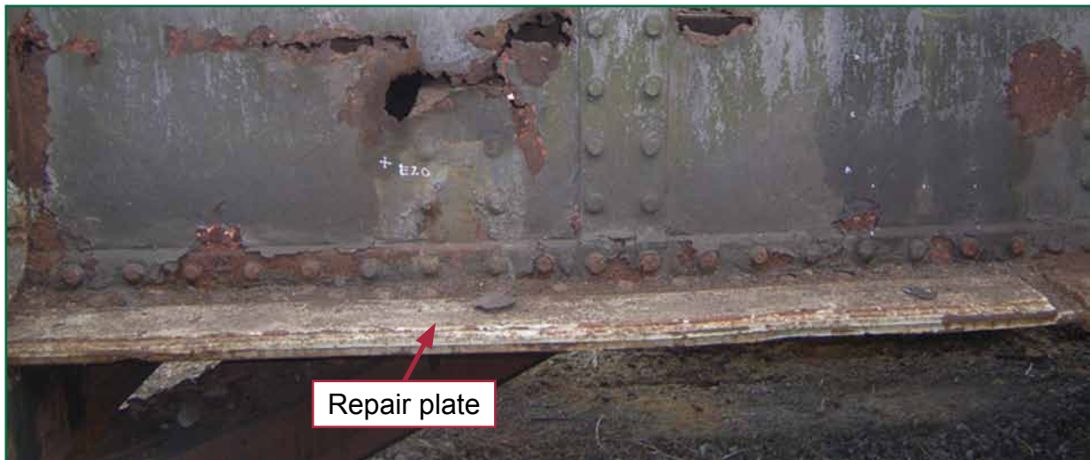
Figure F2: Repair to bottom flange of the east main girder
