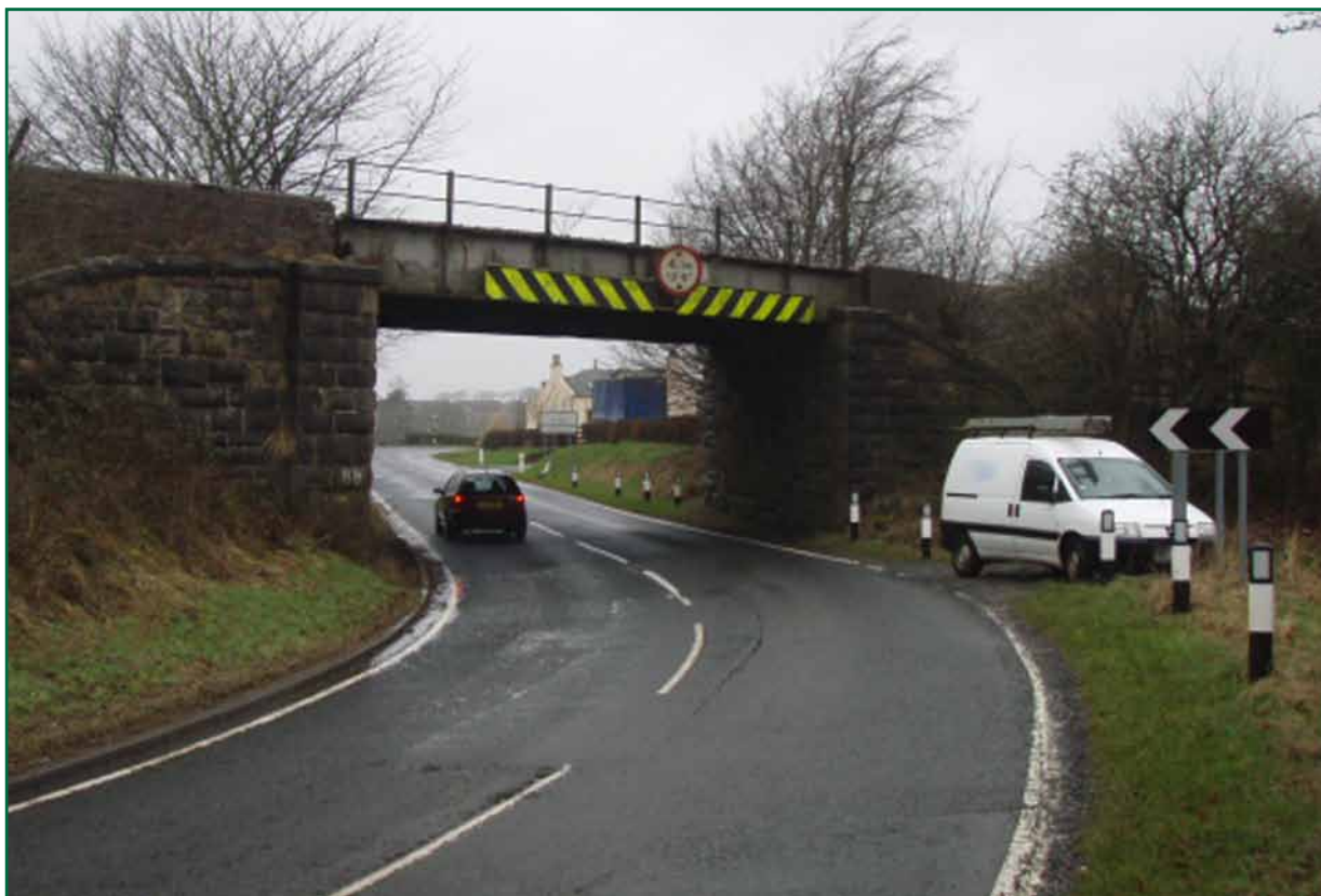
Figure 6: East elevation of Bridge 88 in February 2008 (photograph courtesy of Network Rail)
