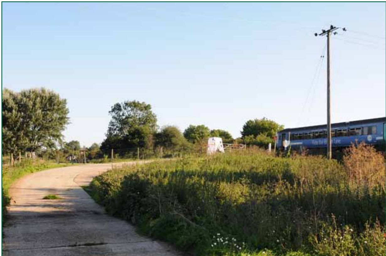
Figure 7: View of the crossing from the exit of the sewage treatment works.
