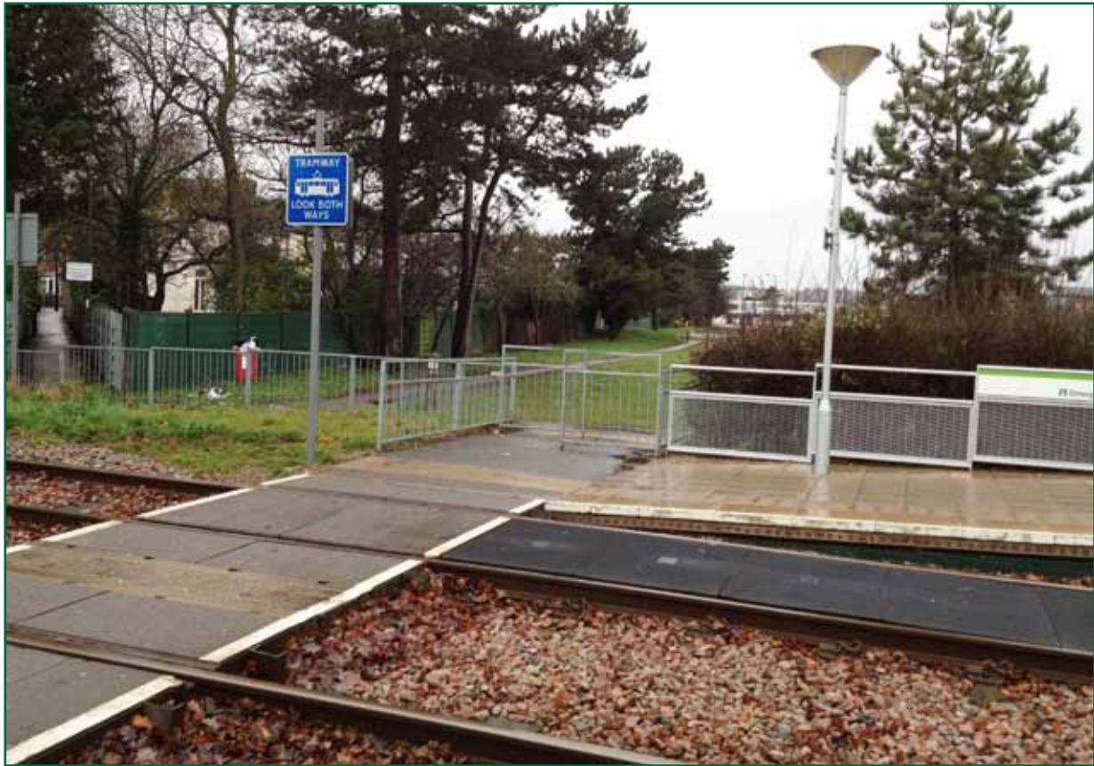
Figure 6: Barriers installed at Arena tram stop
