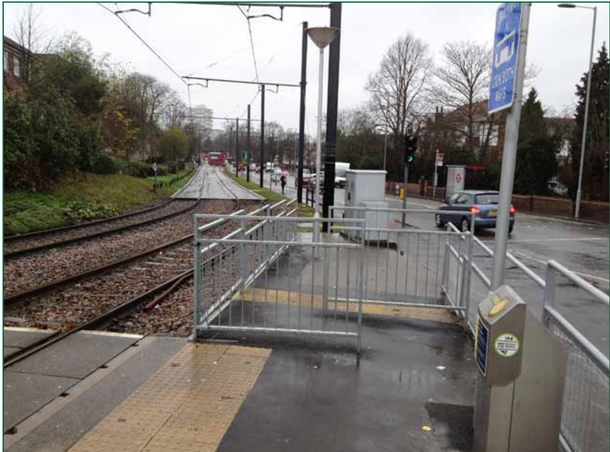
Figure 9: Revised arrangements for pedestrians, including a chicane, at the west end of the eastbound platform at Sandilands tram stop
