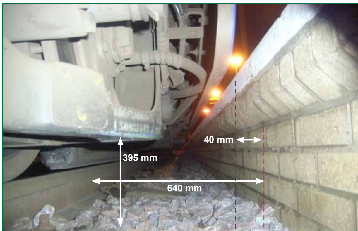
Figure 8: Key dimensions in the gap between the platform face, platform-side rail and a tram
