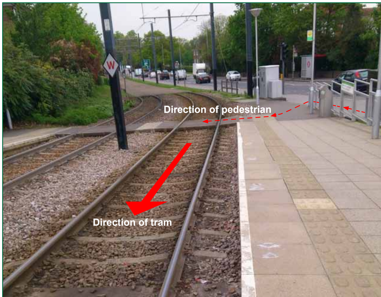
Figure 2: Sandilands tram stop showing the crossing at the west end where the accident happened
