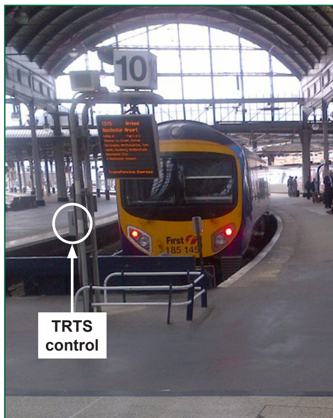
Figure 6: Platform 10 TRTS control (Image courtesy of First TransPennine Express)
