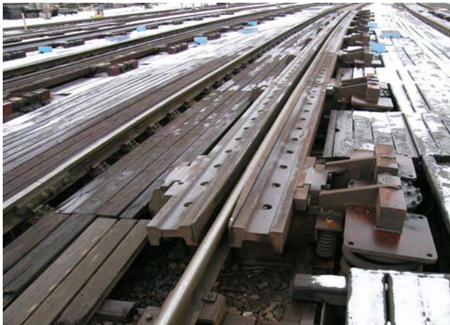
Figure 4: The mechanical brake is a beam brake that pinches against the rail car wheel.
