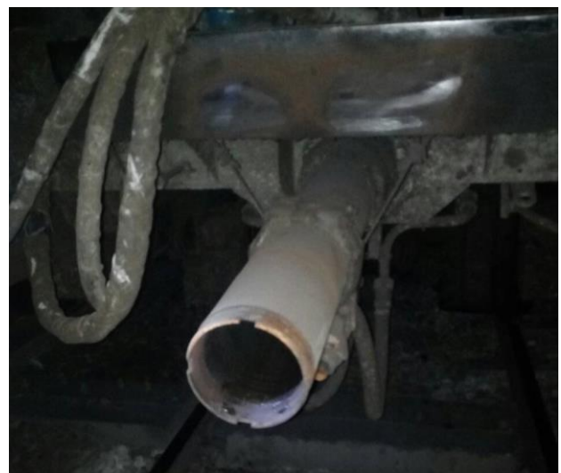
Figure 3.4.4.2: Appearance of a part of the decoupled coupling on the power car 412-061
