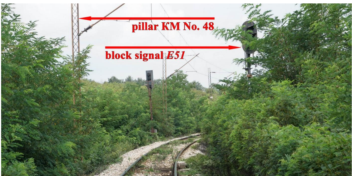
Figure 3.4.2.2: Position of the automatic block signal E 51 opposite the pillar KM No. 48
