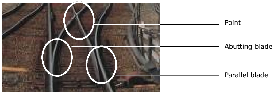
Figure 8 - Switch without movable point
