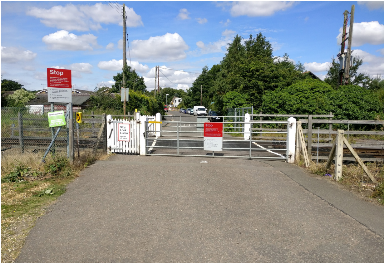
Figure 4: Dock Lane user worked crossing, viewed from river (east) side of railway
