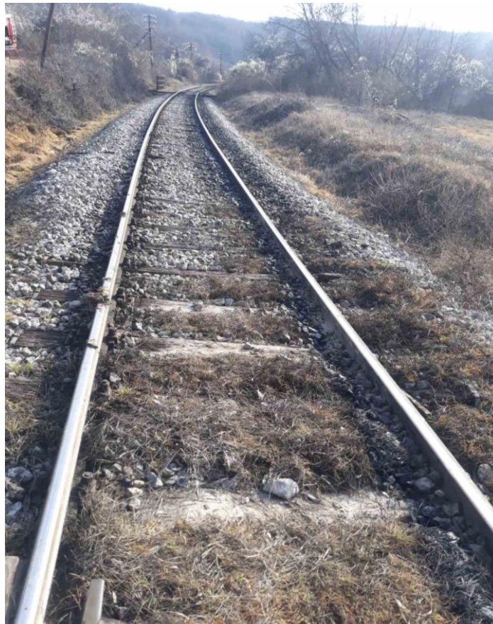
Figure 3.4.2.4: The track grid made of crushed limestone (source: “IŽS” a.d.)
