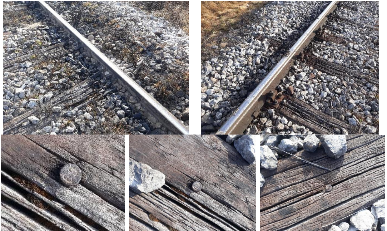
Figure 4.2.9.3: Overview of the sleepers
