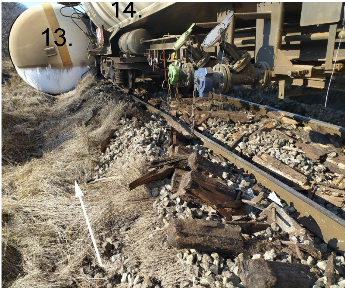
Figure 4.2.1.18: Severely damaged track in the fourteenth wagon area
