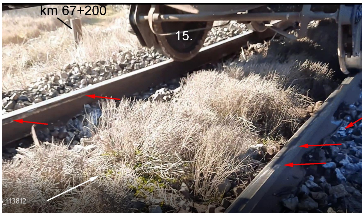
Figure 4.2.1.17: Trace of derailment on the right rail
