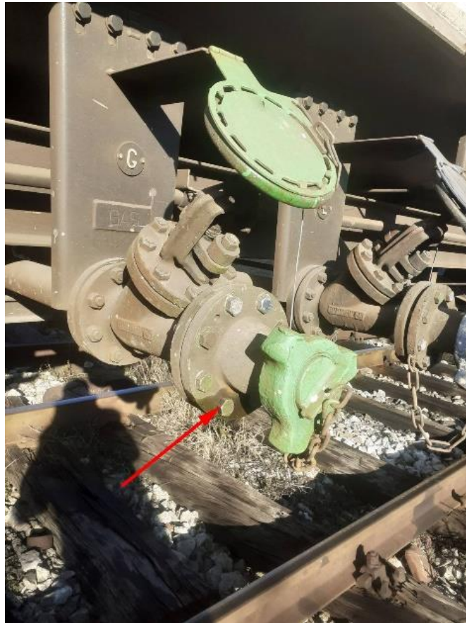
Figure 4.2.5.2.2: The point of ammonia leakage on the eighth wagon-tank No. 33 80 7818 092-8
