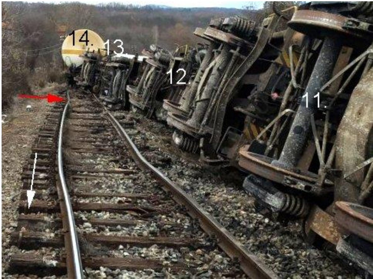
Figure 4.2.1.7: Track deformation in the zone of the front thirteen wagon bogie
