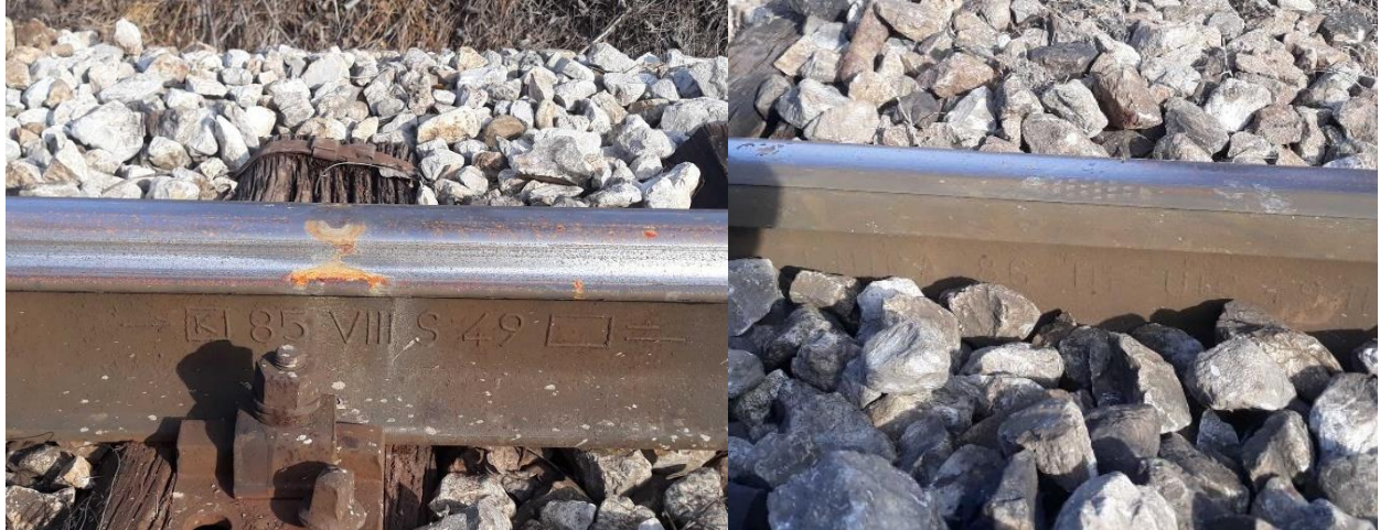
Figure 3.4.2.1: Appearance of the rails type "49E1" ZENICA 85 and 86 UIC 49 (source: "IŽS" a.d.)
