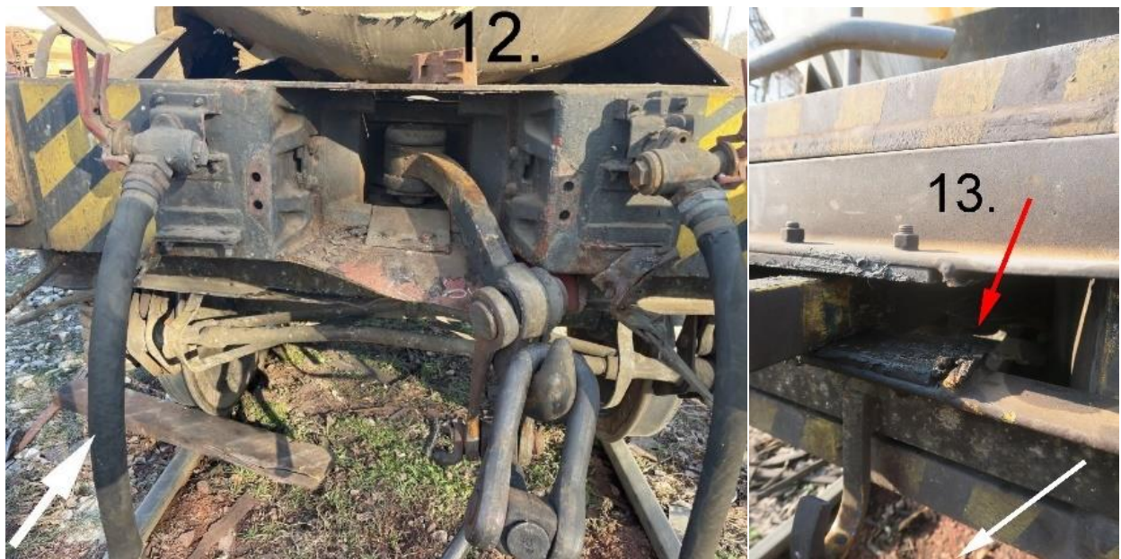
Figure 4.2.1.6: Deformed hooks and guides between the twelfth and thirteenth wagon
