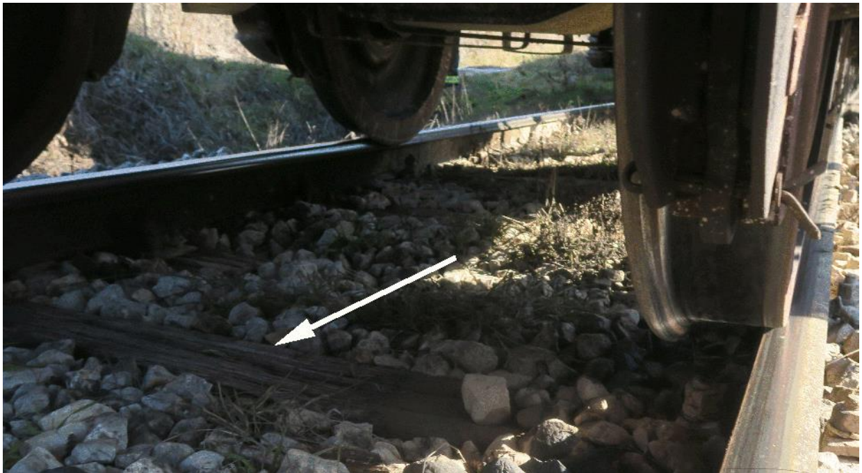
Figure 4.2.1.15: Position on the rail of the third axle of the seventeenth wagon's left wheel
