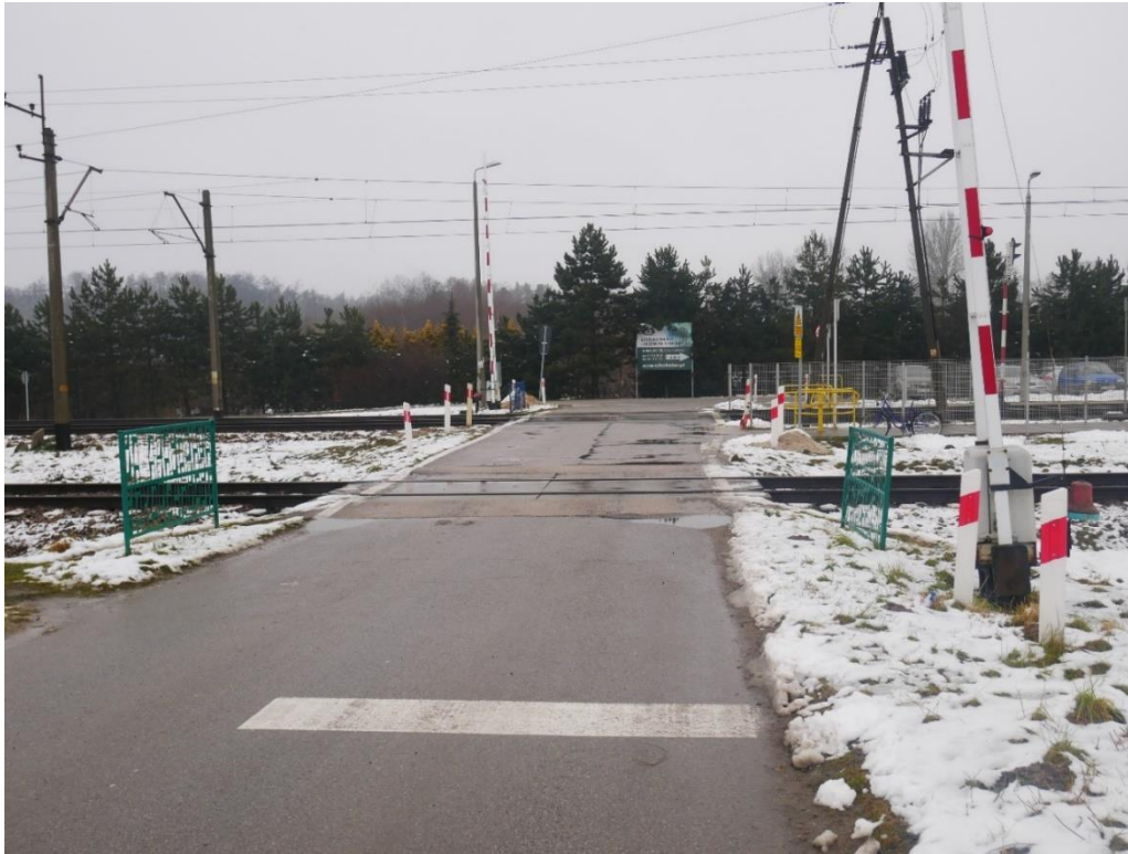
Photo 9 - View of the Cat A crossing km 244.630 with fencing (PKBWK's own material).
