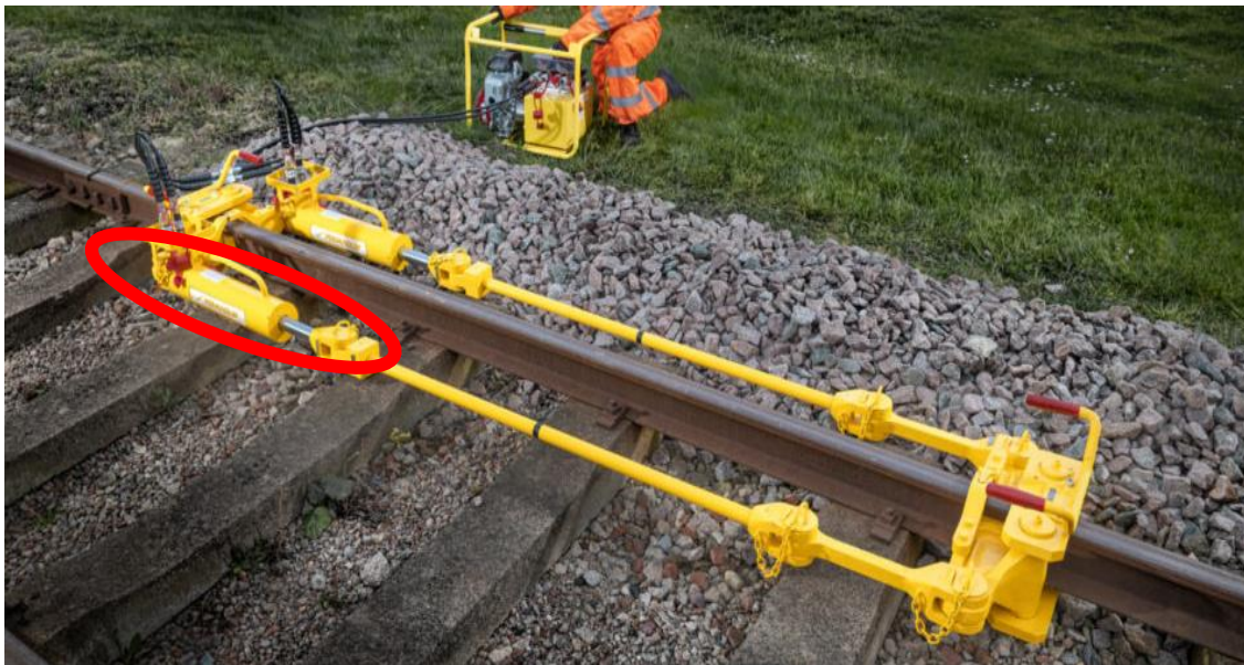
Figure 5 – Rail Tensors attached to rail
